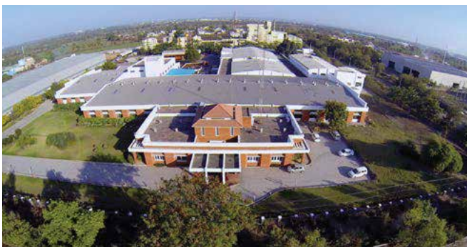
Johnson lifts factory, Nagpur
