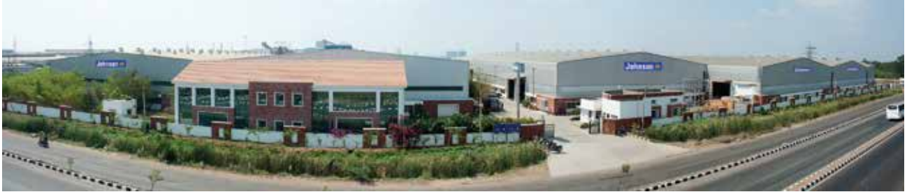
Escalator factory complex in Oragadam, Chennai
