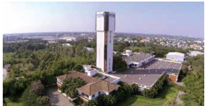
Lift factory in Poonamallee, Chennai
