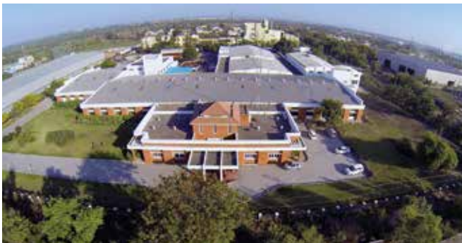
Lift factory, Nagpur
