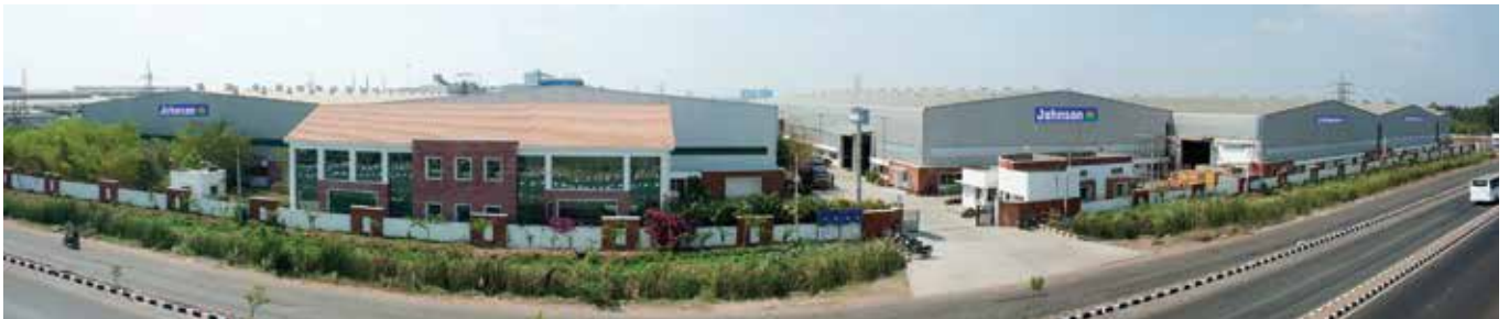
Escalator factory complex in Oragadam, Chennai
