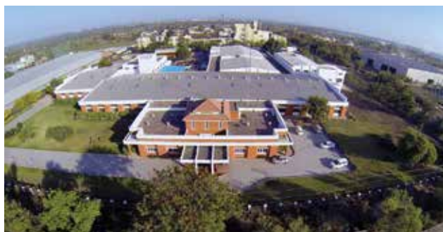
Lift factory, Nagpur
