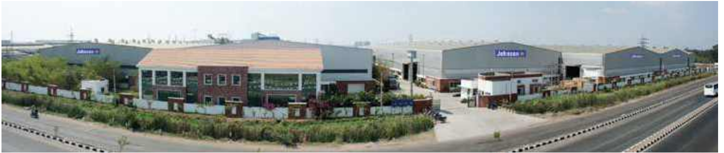
Escalator factory complex in Oragadam, Chennai
