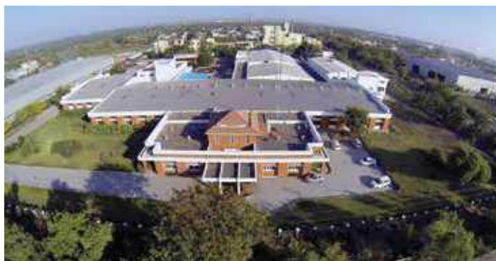
Lift factory, Nagpur
