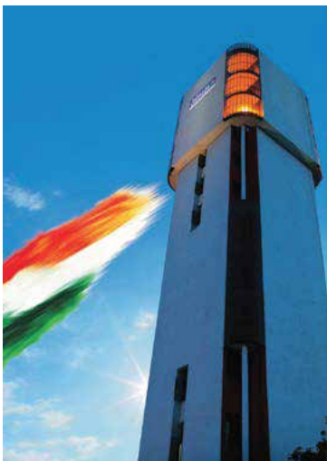
At 155 feet, one of the tallest lift testing towers in India at our Chennai factory.
