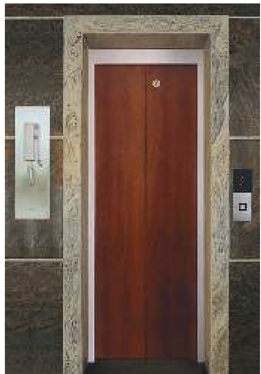
Compact Logix Control Panel fitted on front fascia of the top landing.
