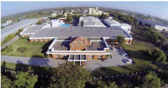
Lift factory, Nagpur
