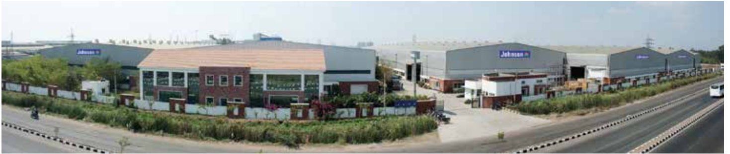
Escalator factory complex in Oragadam, Chennai
